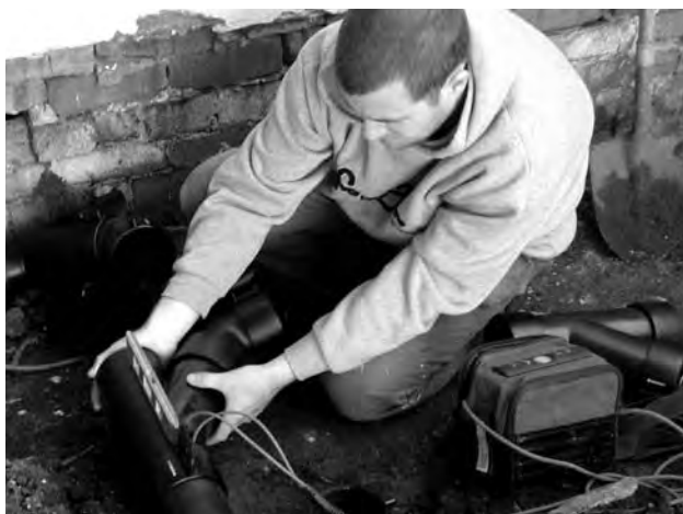
WORKING WITH ‘GREENER’ PLUMBING MATERIALS
